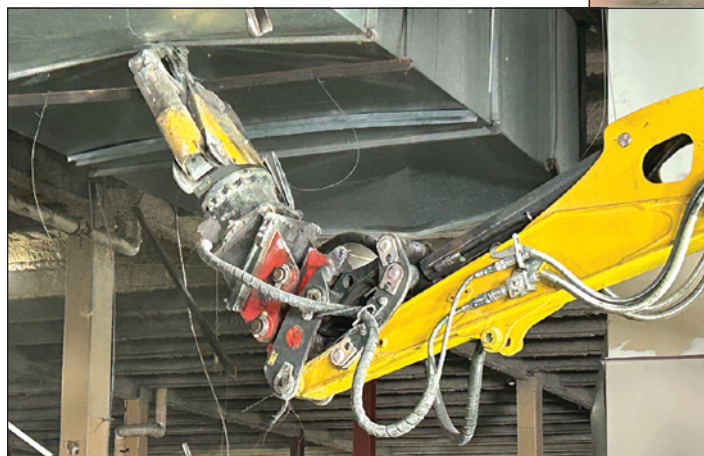
The DARDA shear/crusher attachment with interchangeable heads and a pressure-boosting concept allows high power on smaller carriers.
